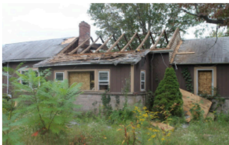
Open rafter sets mark where Jonathan Wuerth extricated the original timber frame of the schoolhouse.
