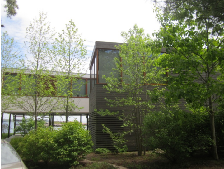
West view (camera facing east)
