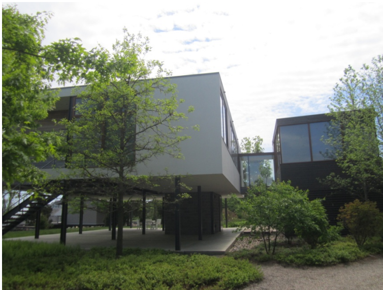
North view (camera facing south)
