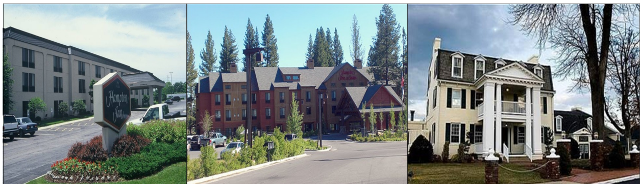
At left is the typical design of a Hampton Inn. Pictured center is a Hampton Inn in Truckee, California and on the right is a Hampton Inn in Leesburg, Virginia. Both are designed to complement their community’s character.
