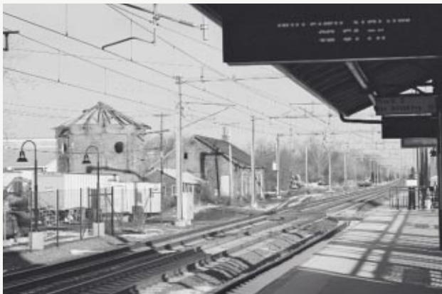
ACROSS THE TRACKS FROM GUILFORD’S NEW TRAIN STATION SURVIVORS OF THE AGE OF STEAM LOCOMOTION AWAIT RESTORATION AND REUSE. PHOTO BY ELLEN EBERT
