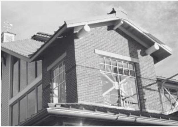
GUILFORD'S NEW UP-AND-OVER TRAIN STATION PROMISES TO BE A FOCUS OF RAIL-ORIENTED DEVELOPMENT. PHOTO BY ELLEN EBERT
