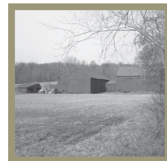
Barn complex at 1592 West Street
