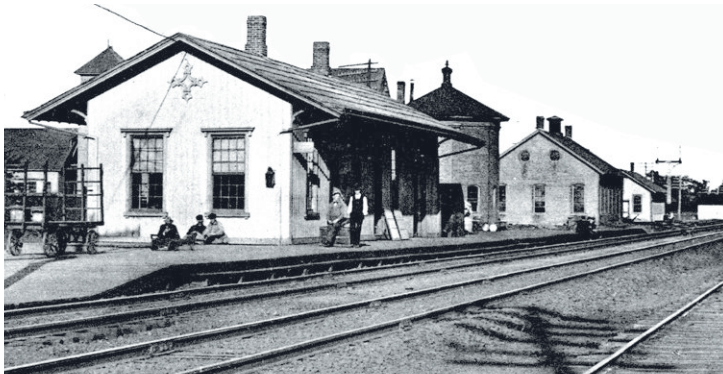
THE 125 YEAR-OLD GUILFORD DEPOT (FOREGROUND) WAS DEMOLISHED BY AMTRAK WITHOUT WARNING ON FEB. 23, 2003.
